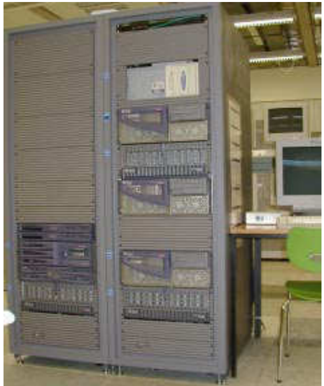
Sun-Server in Rackmontage
